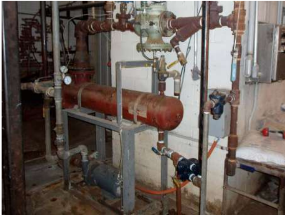
Blowdown / Make up Water Heat Exchanger
